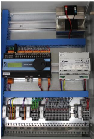
VOICE *agent* modules were installed in all the properties for local data capture. The connection via the Internet served as the primary communication path, while the installed LTE modem served as a back-up in the event of a failure.
