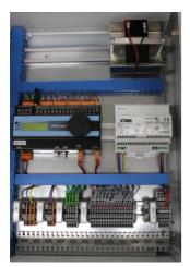
VOICE agent modules were installed in all the properties for local data capture. The connection via the Internet served as the primary communication path, while the installed LTE modem served as a back-up in the event of a failure.
